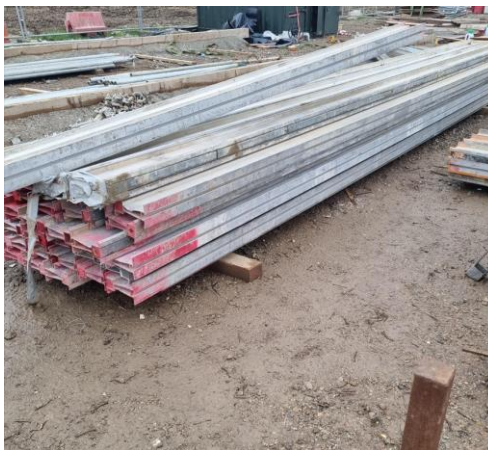
Materials being stacked at time of injury
