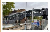
To facilitate the proposed footbridge, the canopies need to be partially demolished to fit in the new footbridge. The existing footbridge and ticket office will remain in service during construction and will be decommissioned and demolished once the new structure is commissioned. This is because it will provide a means of entry to the station and platforms for passengers throughout the construction phase until the new footbridge is fully functional.
