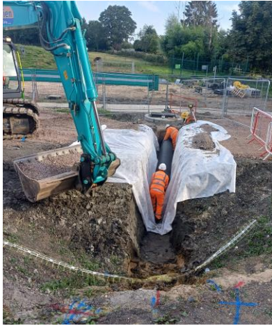
Operatives working in an unsupported excavation
