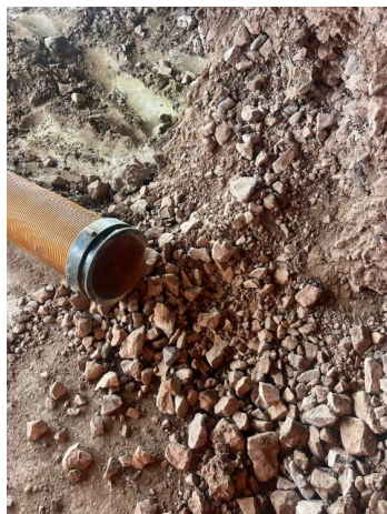
Vacuum Excavator Hose.
