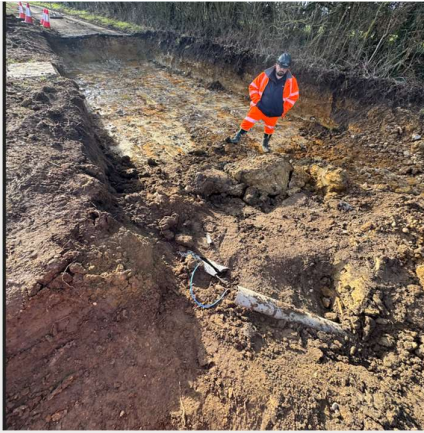
Location of service strike with chamber adjacent.
