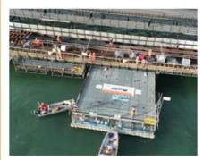
Installation of Monoflex on the cess side of the operational track to protect public from over spray from jet washing.
